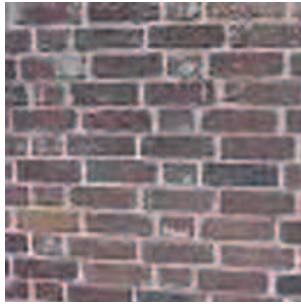
Flemish Bonded and English Bonded brickwork
