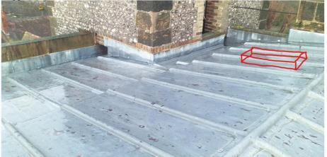
• To keep the lid to a manageable weight, we suggest code 5 lead. The new lead upstand is to be insitu welded to the existing roof lead, which will require a "Hot Works Permit" and the insurance company may insist on a dedicated "Fire Watcher."
