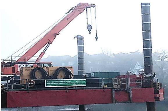
The jack-up barge in Arundel for working in water environments.
